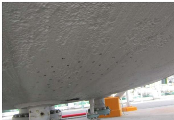
**Figure 5: Corrosion at the bottom of pressure vessel**
